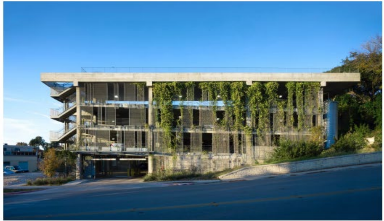
T3 Parking Structure, Austin, TX • Living Vegetation Facade
