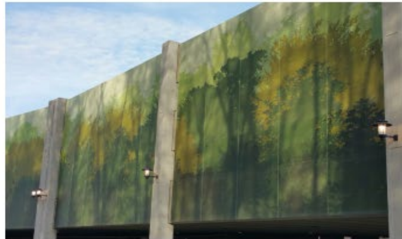
Crocker Park Parking Garage, Westlake, OH • Tensile Mesh Facade, Custom Printed with Tree Pattern Image
